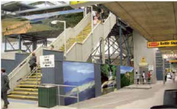
EXAMPLE OF HOARDINGS WITHIN A PUBLIC SPACE UNDER CONSTRUCTION
