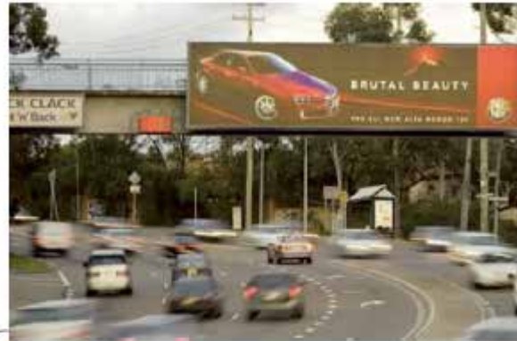
PROTRUDES ABOVE THE TOP OF THE ROAD BRIDGE; NOT IN KEEPING WITH BRIDGE ARCHITECTURE
