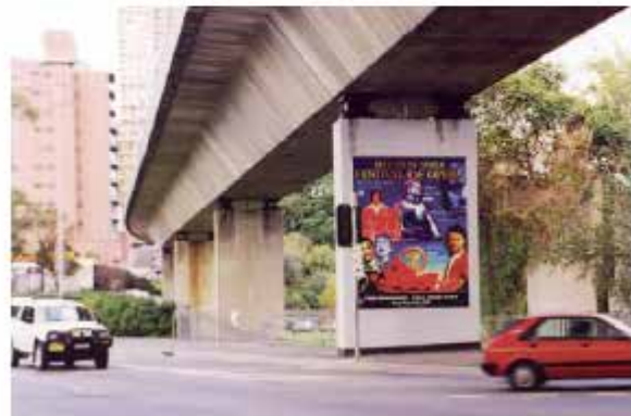
ADVERTISEMENT WITHIN STRUCTURAL BOUNDARIES OF RAIL BRIDGE
